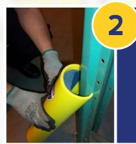
Slide one edge of the top of the Rack Armour® guard around the side of the frame/upright so that the edge of the guard hooks behind the frame profile.
