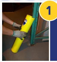
Tilt the Rack Armour<sup>®</sup> guard forward so that the bottom of the unit is approximately 300mm clear of the upright and hold at an angle of 45 degrees.
