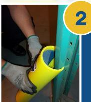
Slide one edge of the top of the Rack Armour® guard around the side of the frame/upright so that the edge of the guard hooks behind the frame profile.
