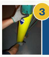
Ensure the top of the guard has clipped into place.
